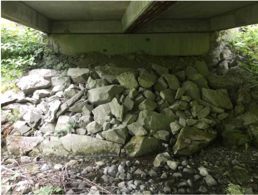
Right Bank Abutment when facing downstream
