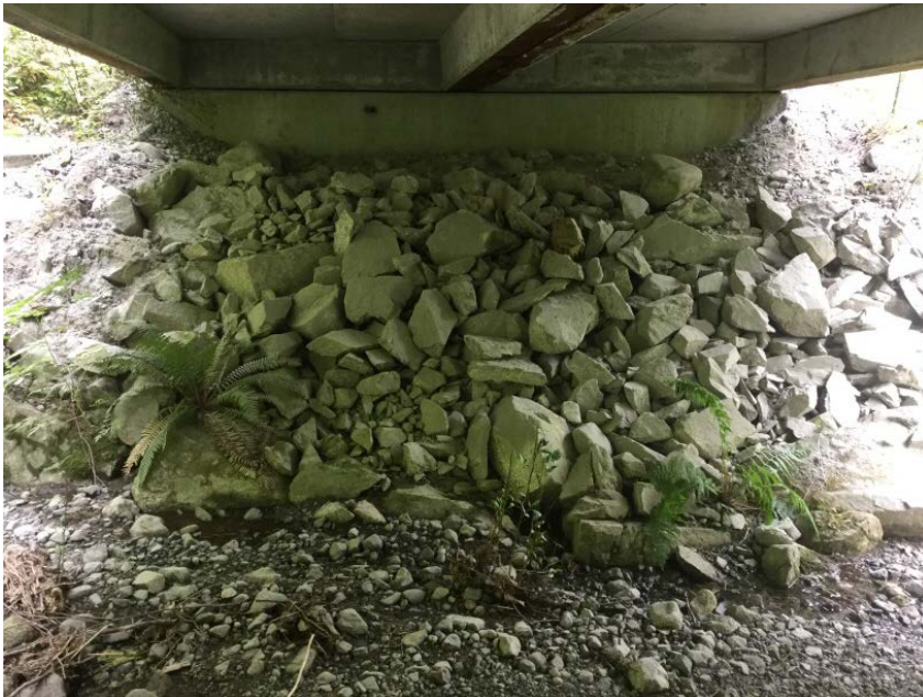
Left Bank Abutment when facing downstream
